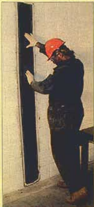
Figure 1. Applying vertical strap to reinforce masonry wall.
